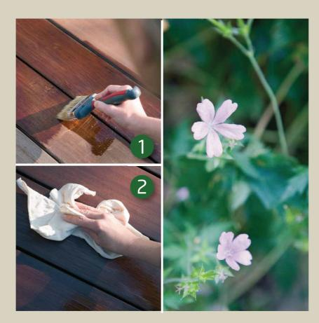
Exterior Oil, Exclusive to be used outdoor for basic treatment and maintenance of new and previously oiled wood surfaces such as decks, garden furniture, cladding etc.
